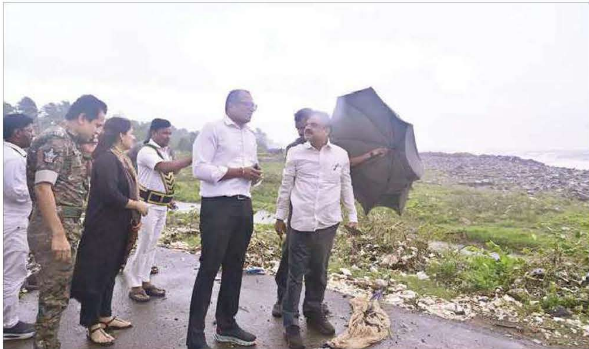
Collector MN Harendhira Prasad visiting Uppada beach road which was damaged by the cyclone
