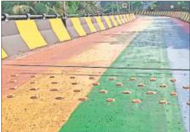
Cat’s eye reflectors were installed on Kolkata flyover, Thursday. EXPRESS
