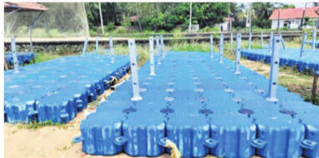
Floating bridge that stretched into the sea lies idle on shore | EXPRESS
