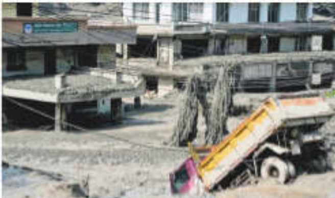
Damaged houses and vehicles are seen in the aftermath of flash floods along the Trishuli River in Nepal's Nuwakot district on Wednesday | AP
